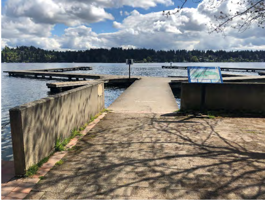
Photograph 3. Looking east from plaza over existing docks (April 2021).
